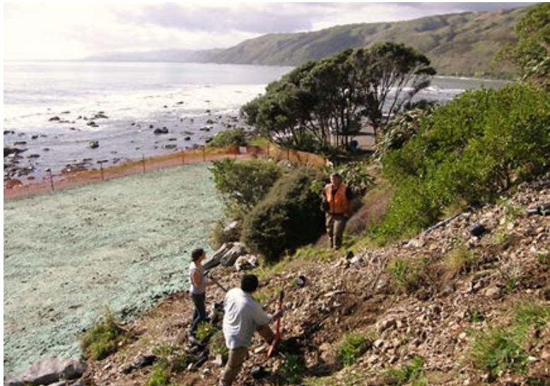
Turning concrete into paradise – 70 volunteers planted 1500 shrubs with PCC staff
